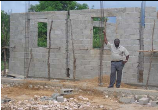
Caleb stands on our new front porch! Estimated completion summer 2007
